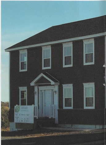
The EcoPlusHome boasts triple-glazed, low-E krypton gas windows.
