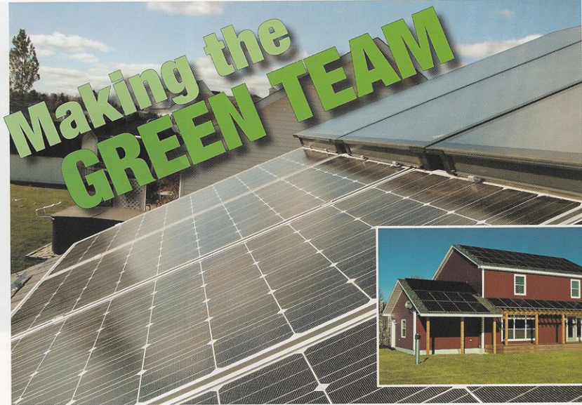
Photovoltaic panels and a solar thermal system are among the features of the EcoPlusHome. Photos courtesy Tight Lines Productions Ltd.
